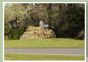
Construction work: parking and storing of materials
