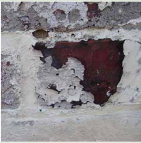
◀ Gloss paints are plastic based. Once cracked these paints can hold moisture against the surface of the masonry.
