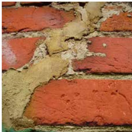
Example of poor repointing using cement mortar which not only looks unsightly but will damage the brickwork in the long term
