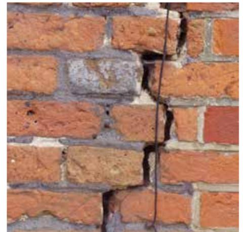
Vertical crack in brickwork due to movement. Brickwork has been repaired with a variety of hard mortars which have failed to address the problems
