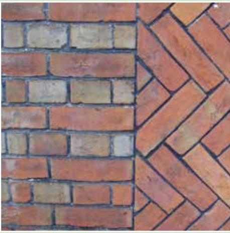
Think carefully whether any repointing is really necessary. This brickwork and mortar is perfectly sound. The joints are full, the lime mortar is taking and expelling moisture effectively and the character of the wall is intact
