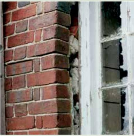
◀ Bulging has occurred here. Subsidence and the corroding iron wall ties have allowed the outer leaf of brickwork to bow outwards
