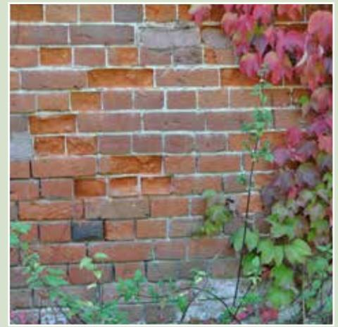
Poor repairs and damage caused to brickwork due to the use of cement mortar
