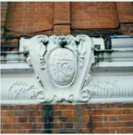
◀ The cornice has created a splash back against the brickwork. It is consequently staining and eroding the brick above and below the cornice dripping water is also staining the brickwork
