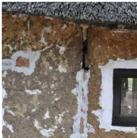
Cob repairs
