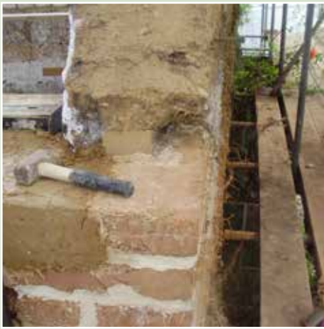
Cob repairs in progress
