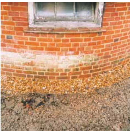
Land drain back-filled with shingle
