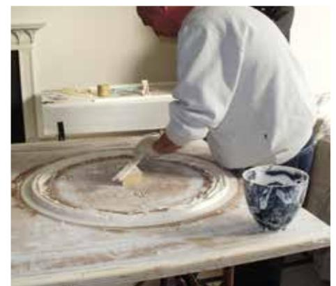
Constructing plasterwork moulding for a moulded ceiling rose
