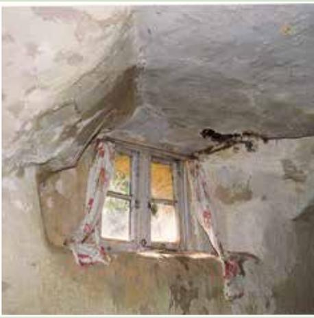
◀ This patched ceiling and wall plaster continues to be affected by damp, as the cause of the problem has not been rectified
