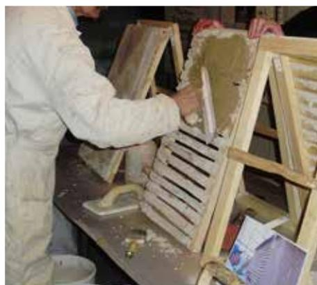
Demonstration showing lime plastering onto lath
